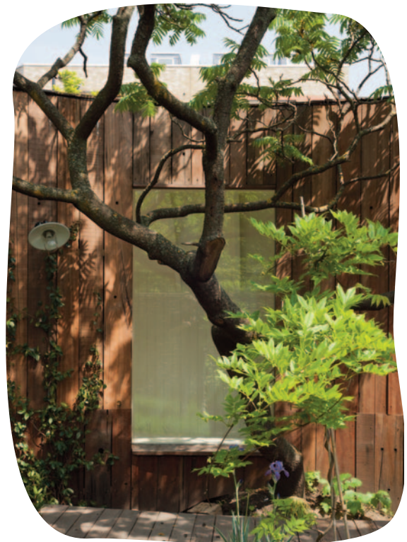
Tree House by 6a architects with reclaimed jarrah cladding from Salvo Code member, Ashwells Reclaimed Timber.
